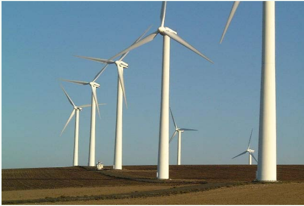
Stateline, Oregon, wind turbines
